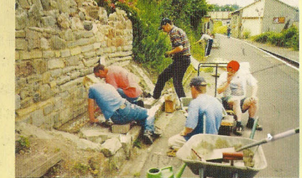
Members of the Seahorse Centre Team working on the Wall
