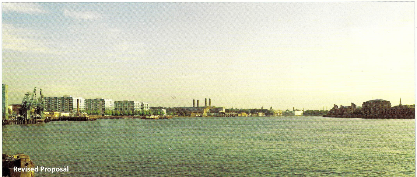
View from the river looking upstream, the removal of the towers makes a significant difference.
